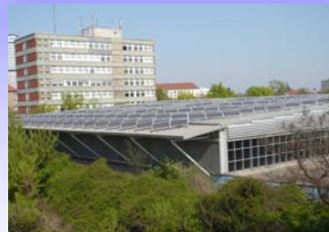
Sporthalle → Kalzip-Dach (60 kW p )
